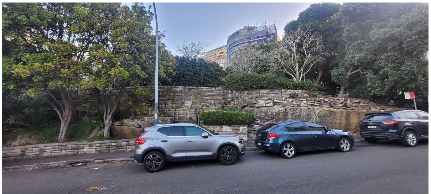
27 View from Billyard Avenue indicating the extensive stonework that was constructed as part of the Berzins plan. Source: Matthew Taylor.
